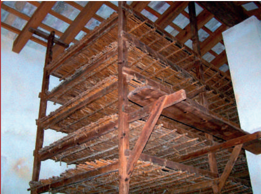
Wooden and wattle structures for silkworm rearing, preserved in the shelf-lined room at Félix Farmhouse
